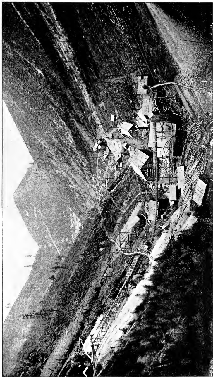
FIG. 98 — View of the Banker Hill and Sullivan Mines, Wardner, Idaho. The vein dips toward the observer, and outcrops on each hill, right and left. From a photograph furnished by E. E. Olcott.
